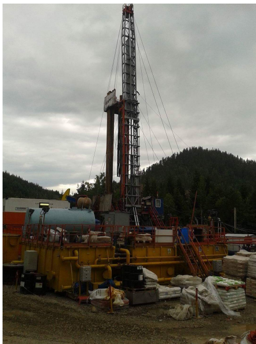
Fig.1 Instalatiya de foraj MR 8000
