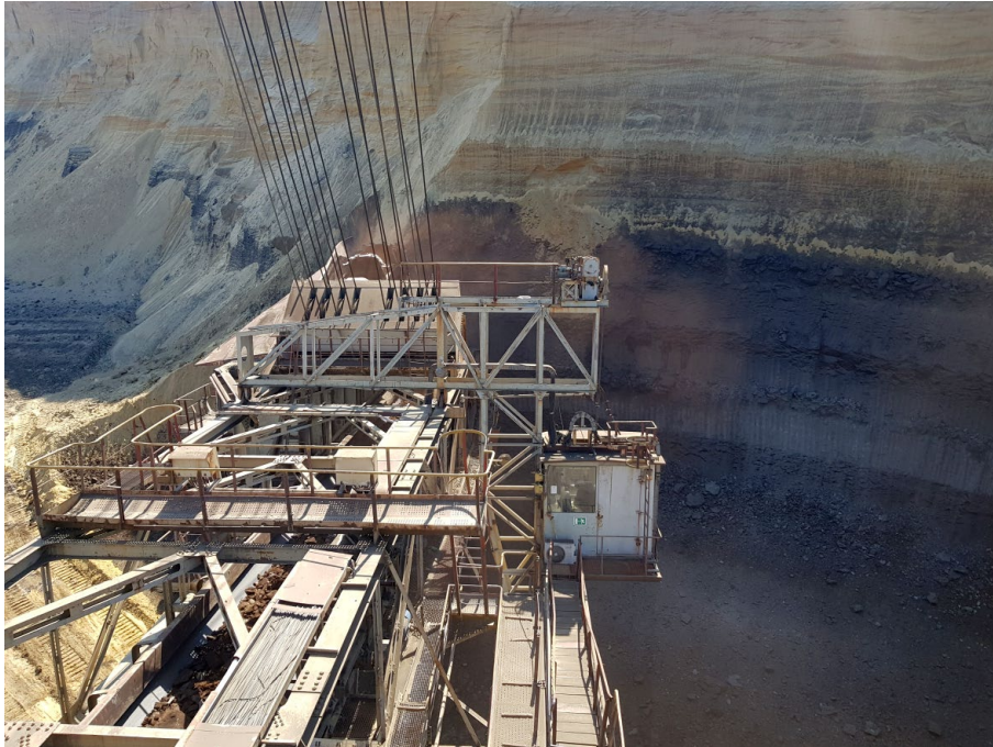
Fig. 2 Earth-marl-coal excavation front
