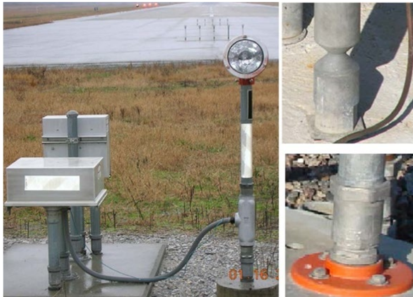
Fig. 1. Examples of frangible couplings.
